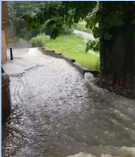
Figure 4 Surface water flowing onto Sites Hill Road
