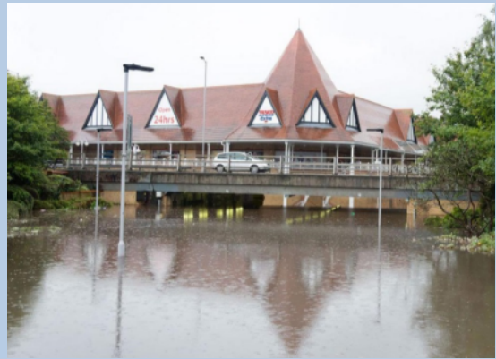
Figure 1 Purley Cross underpass (Croydon,2015)
